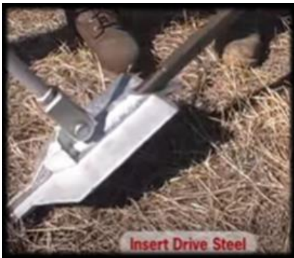
1 Fit the drive steel
